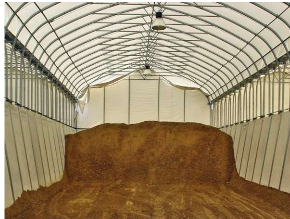
60 000 t contaminated soil excavated, treated and ready for backfill
